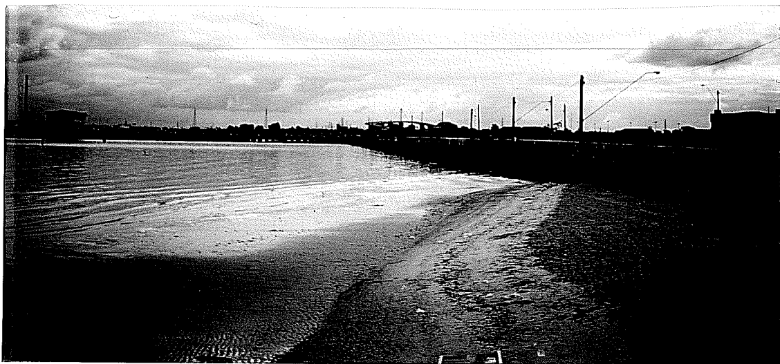
Photo 7. Sea wall to be demolished and replaced with beach.
