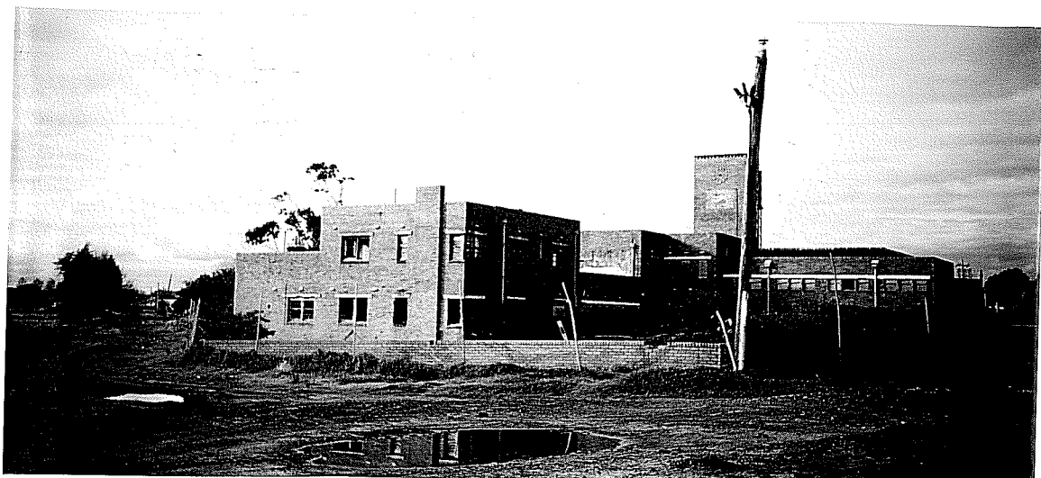
Photo 8. Missions to Seaman's Building
